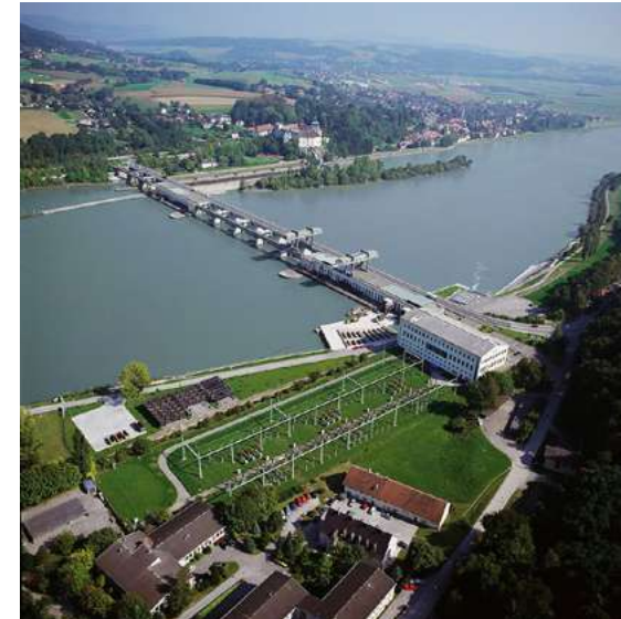
Ybbs-Persenbeug hydroelectric power station. Austria / VERBUND, UWK
